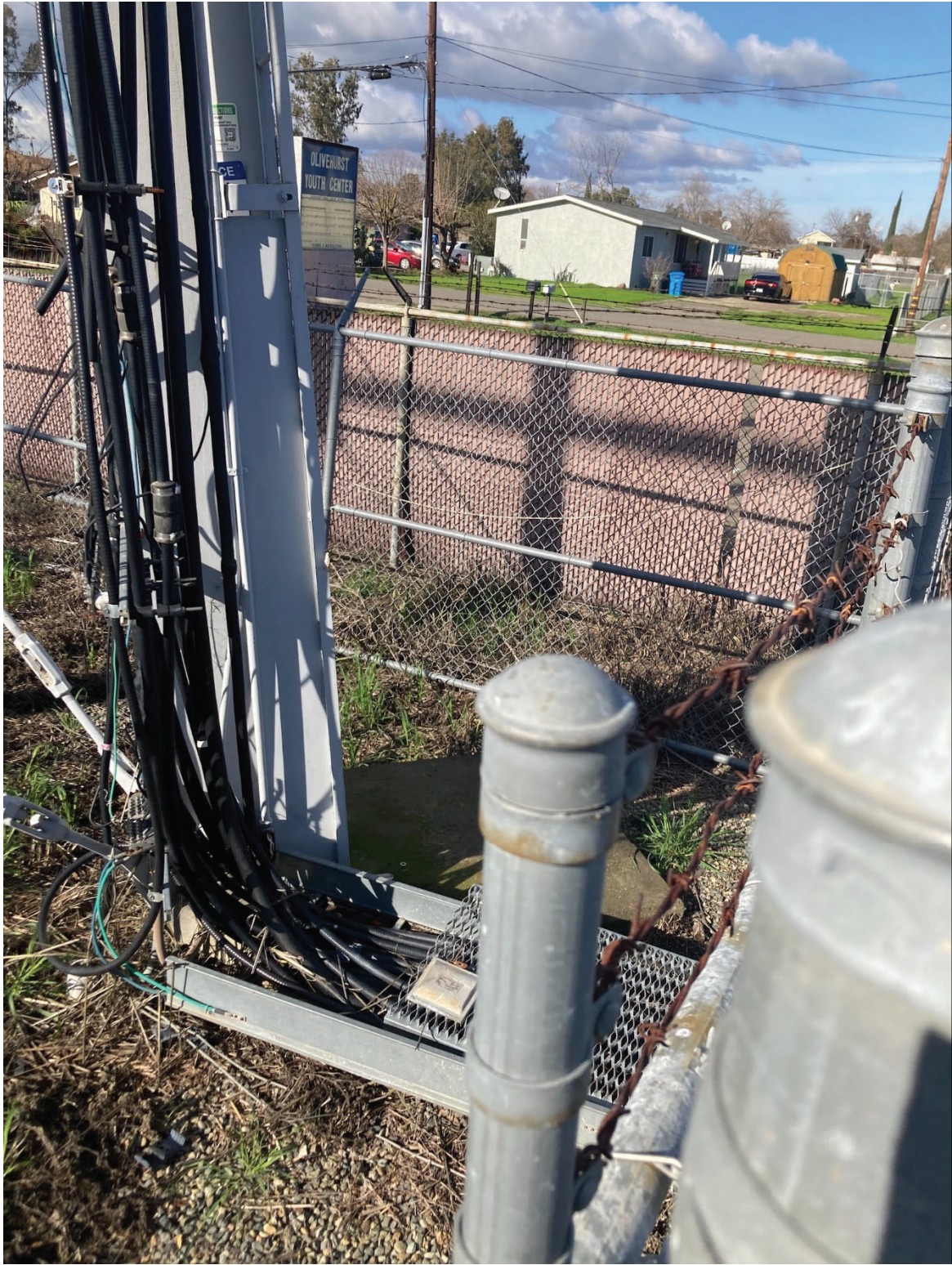
Close Up of Cable Configuration on Tower Leg
