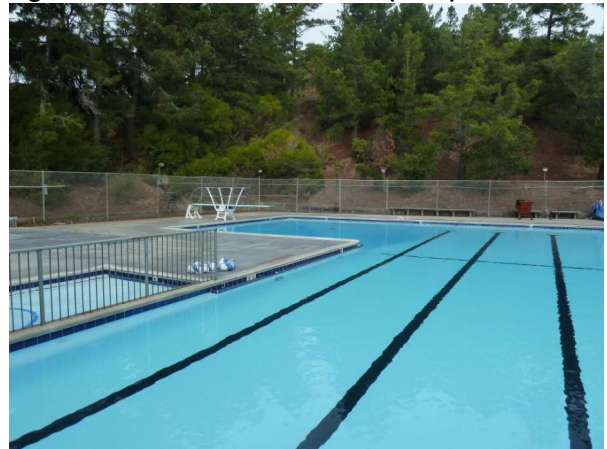
Highlands Recreation District Pool (after)
